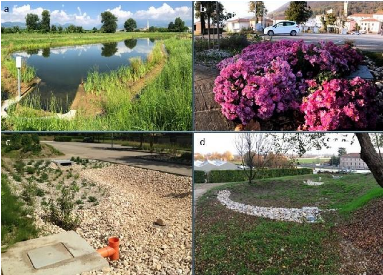
Figure 2.1. Pictures of the interventions monitored by the Action D1 of the BEWARE project: a) water retention basin realized in Giavenale di Schio locality; b) autumn flowering at the intervention of Piazza della Libertà (Santorso); c) the rain garden located in Via dei Prati (Santorso); d) the bioretention area located on the eastern side of the Grumo hill (Santorso).
