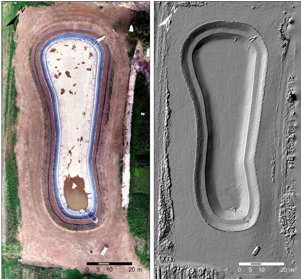
Figure 4.10. Orthophoto mosaic (on the left) and the digital terrain model (hillshade view on the right) obtained by the UAV survey of the empty water retention basin (Action C3).
