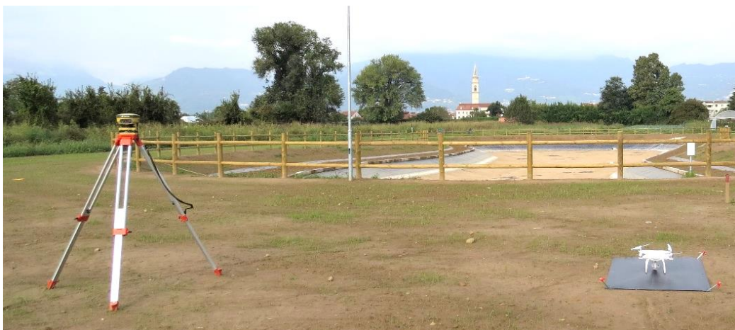
Figure 4.9. Devices used for the high-resolution topographic survey of the empty retention basin (on the background): the DJI Phantom 4 Pro and the Topcon HiPerV differential GPS (used as base station in the picture).
