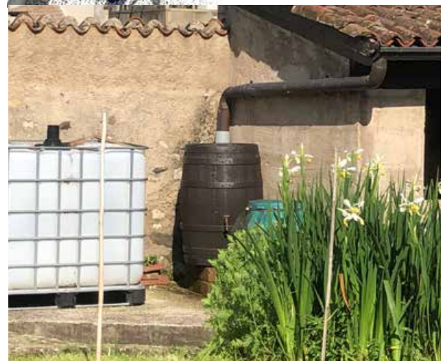
Figure 8: examples of rainwater storage tanks placed above ground at the Corte Acqualiente intervention (for a descriptive video, visit the link https://youtu.be/OwIrip5QYLU ).
