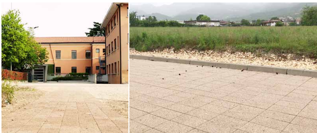
Figure 10: Drainage pavement was constructed as part of the LIFE BEWARE project interventions (further details at the link: https://youtu.be/lARDtC1_kQE ).
