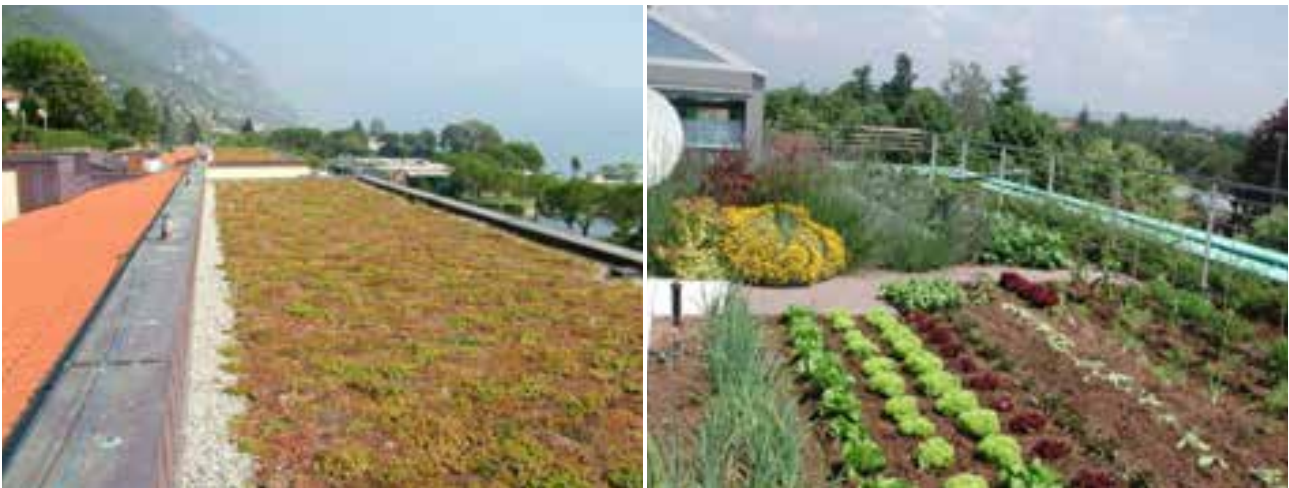
Figure 12: left, extensive type green roofs with Sedum spp., right, intensive type green roofs with vegetable cultivation (source: Andri S., Sauli G., 2012 3 ).
