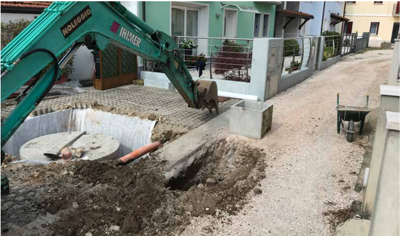
Figure 9: installation of the leaking well carried out within the framework of the LIFE BEWARE project at Corte Aquasaliente (for more pictures of the intervention, watch the video at the link https://youtu.be/Owlrip5QYLU ).
