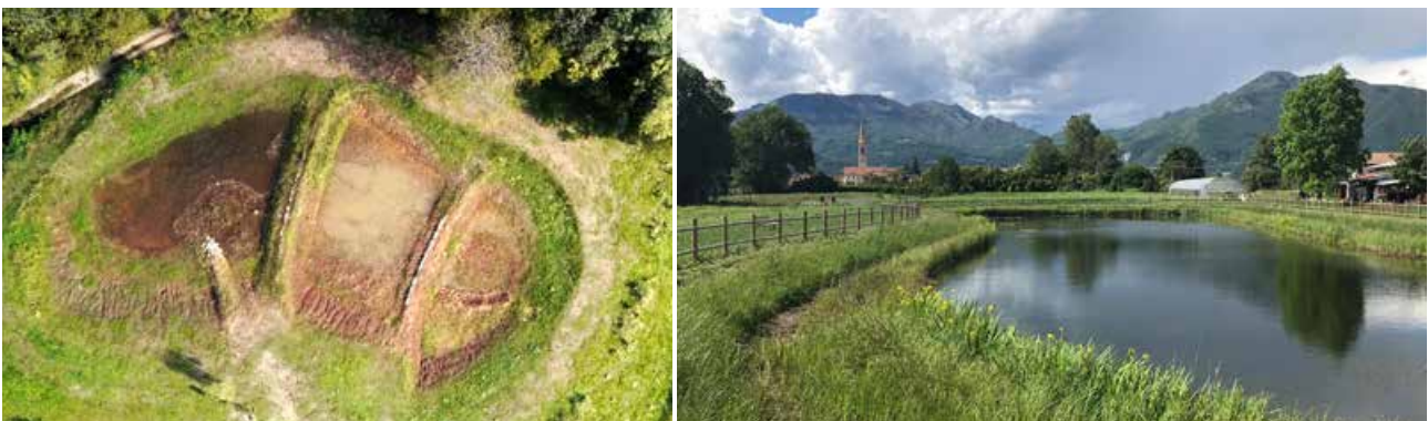
Figure 16: The detention basin with bioretention pond (left - more information at the link https://youtu.be/hVwtT4dlSOI ) and the retention pond (right - more information at the link https://youtu.be/TjrFs7pSojo ) realised within the framework of the LIFE BEWARE project.
