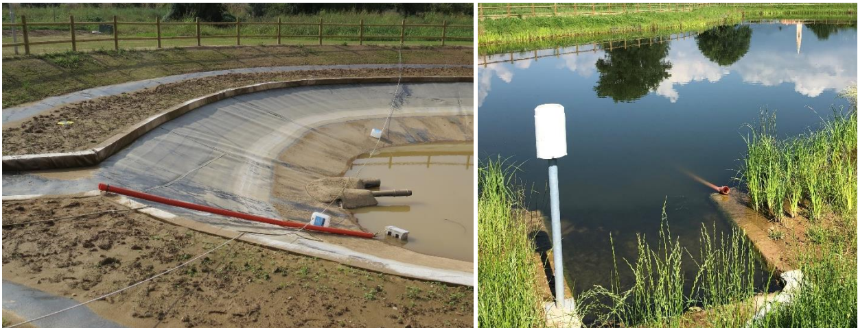
Figure 4.12. The perforated PVC pipe installed on bank of the basin that host the pressure transducer in order to measure the water level.
